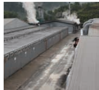
Dry-kiln complex and power plant
